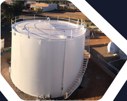
Bulk Storage Tanks
